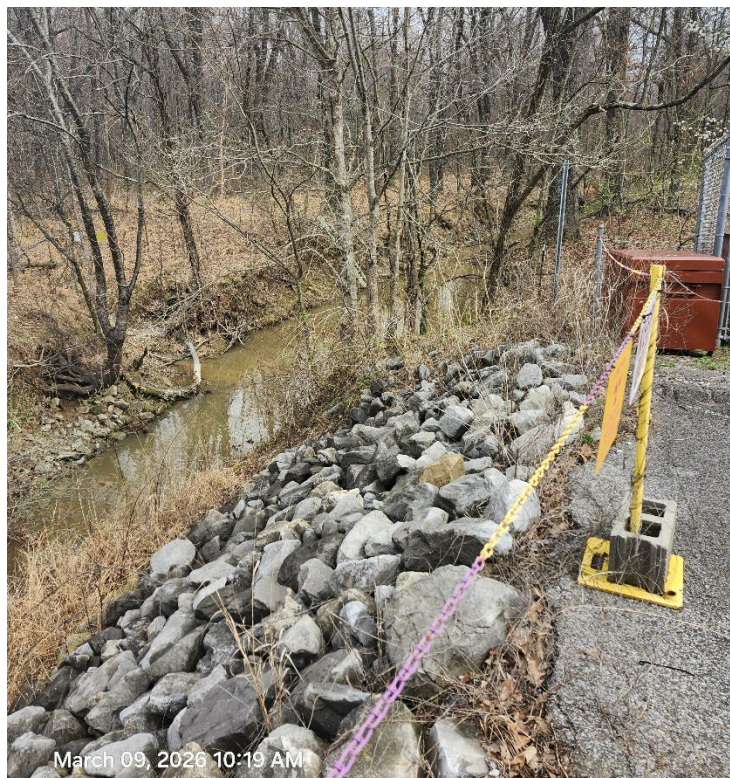
Figure 10. Looking North at Little Bayou Creek—McCaw Road
