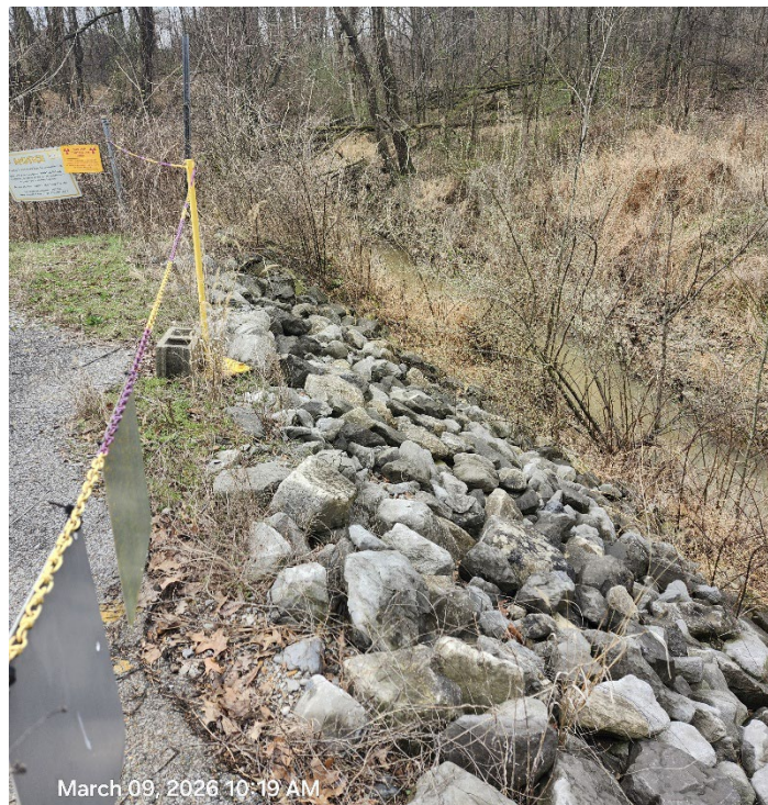
Figure 11. Looking South at Little Bayou Creek—McCaw Road
