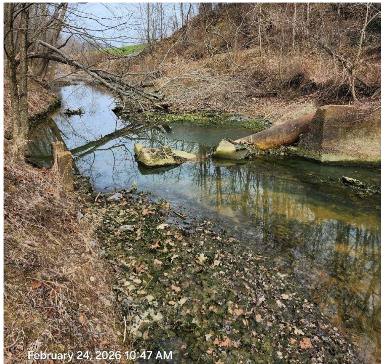
Figure 4. Looking North at Little Bayou Creek— Raw Water Line Crossing on Tennessee Valley Authority (TVA)
