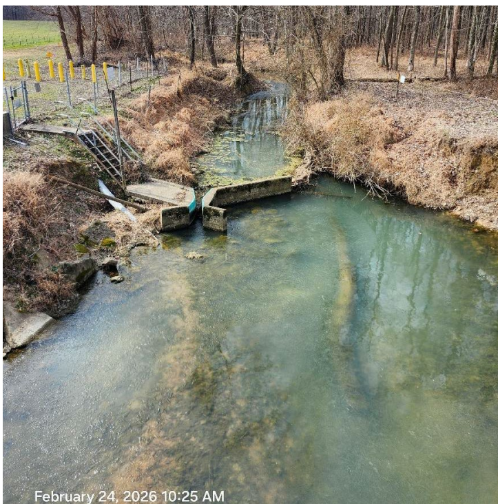
Figure 9. Looking South at Little Bayou Creek— Ogden Landing Road
