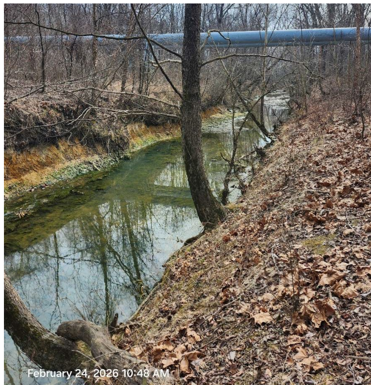
Figure 5. Looking South at Little Bayou Creek— Raw Water Line Crossing on TVA
