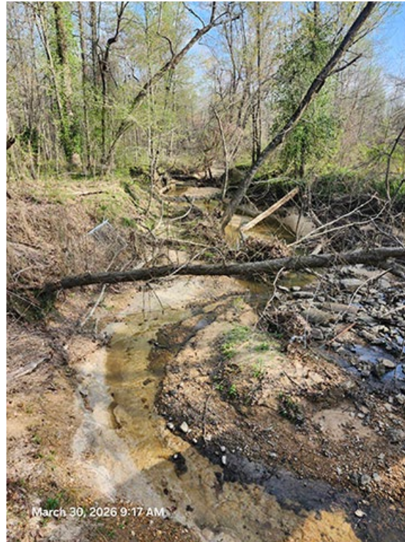
Figure 6. Looking North at Little Bayou Creek—Anderson Road
