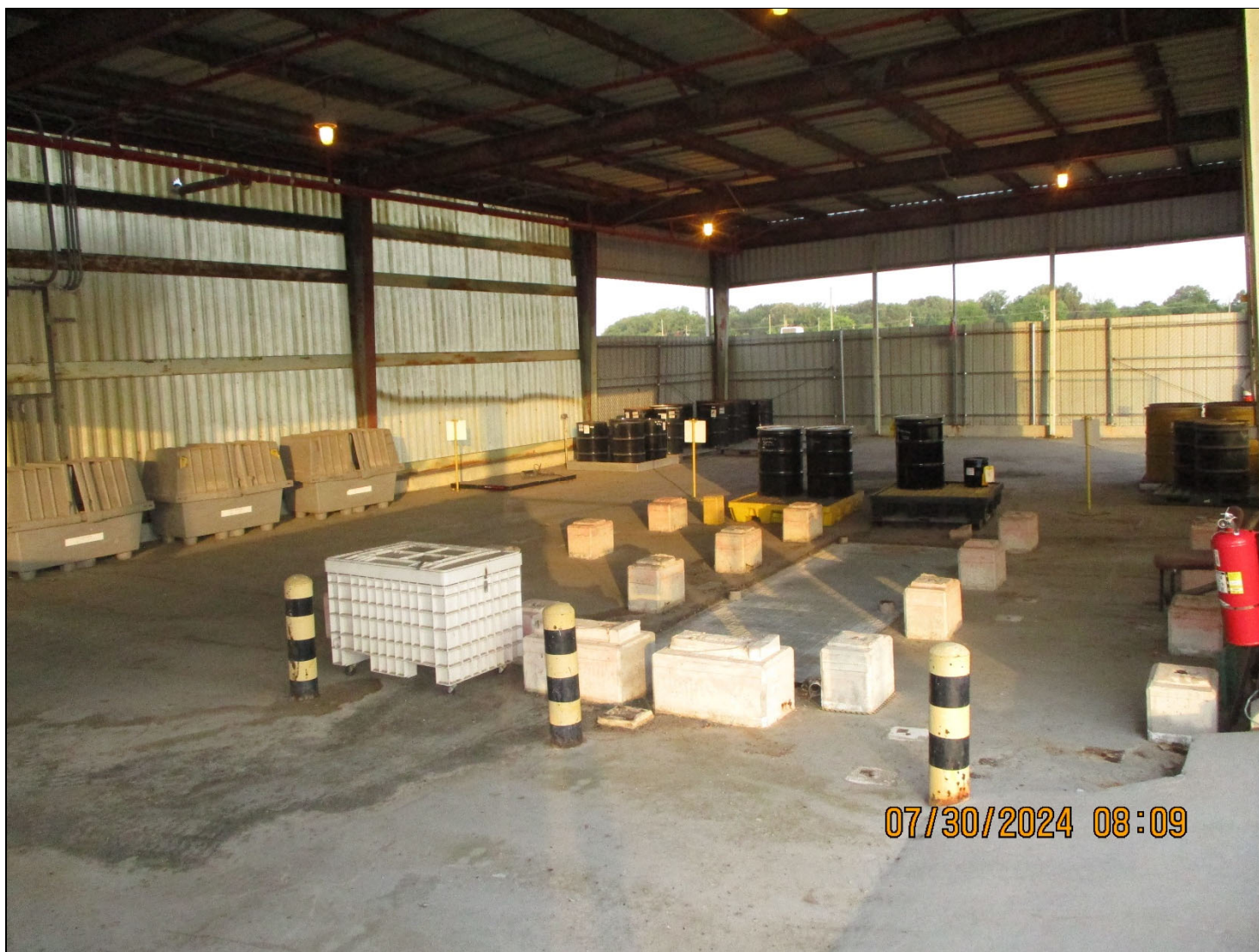
July, 30, 2024 C-733 Hazardous Waste Storage Area (Inside), East Side Facing West Process Codes: S01,T04
