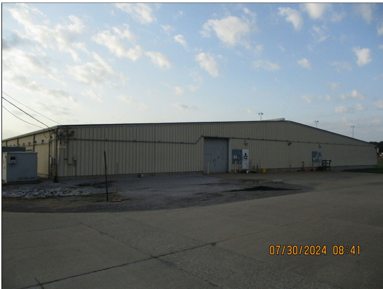
July 30, 2024 C-746-Q Hazardous and Mixed Waste Storage and Treatment Facility (Outside), West Side Facing East Process Codes: S01,T04
