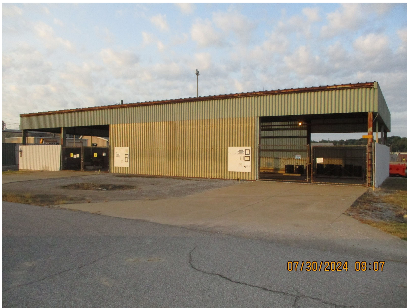
July, 30, 2024 C-733 Hazardous Waste Storage Area (Outside), North Side Facing South Process Codes: S01,T04
