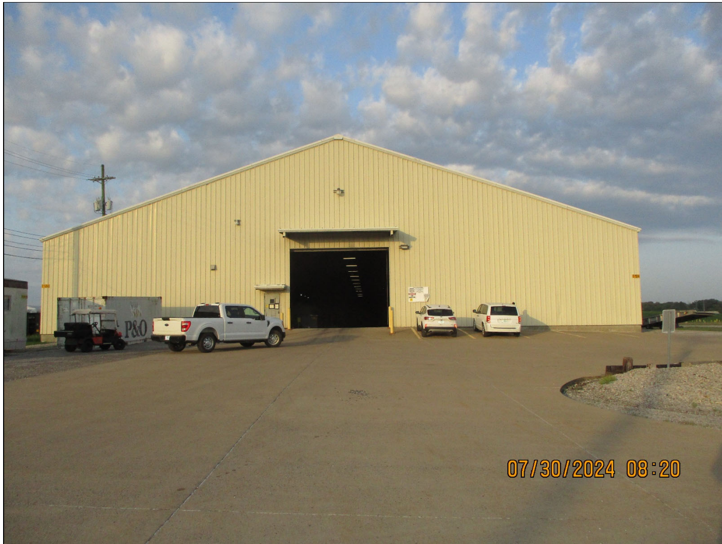
July, 30, 2024 C-752-A Hazardous Waste Storage and Treatment Facility (Outside), North Side Facing South Process Codes: S01,T04
